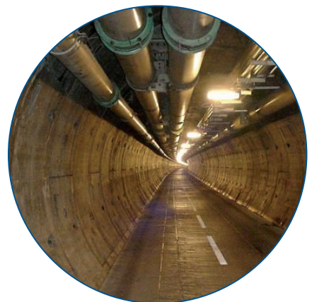
Fig. 6: The service tunnel Photo © Eurotunnel
