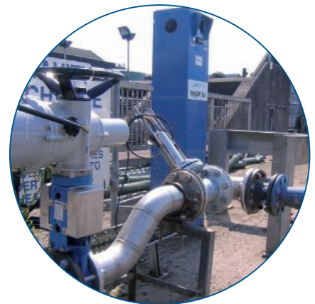
SOLITAX highline sc installed as insertion probe
