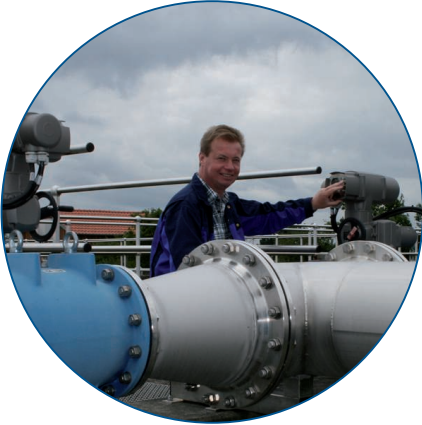
Fig. 3: Operations manager Thomas Hutz regularly checks the new annular piston valves.
