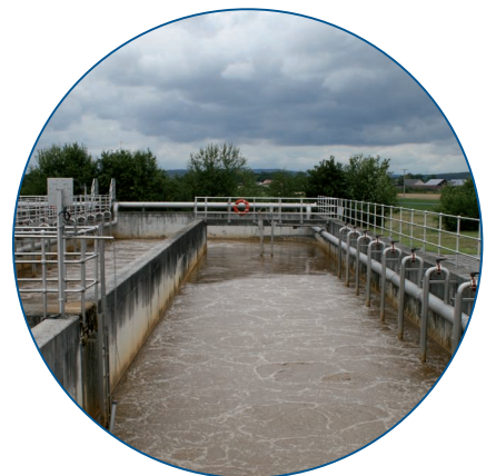
Fig. 2: Aeration tank in Markt Schwarzenfeld.
