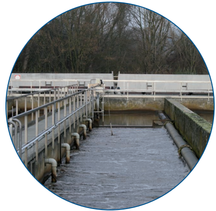
Fig. 4: In future, each channel will have its own targeted carbon supply.
